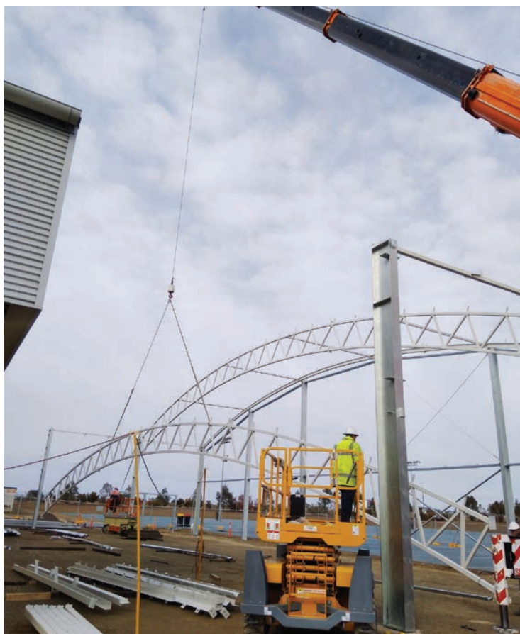
ABOVE: The steel frames for the Sports Dome extension going into place.
