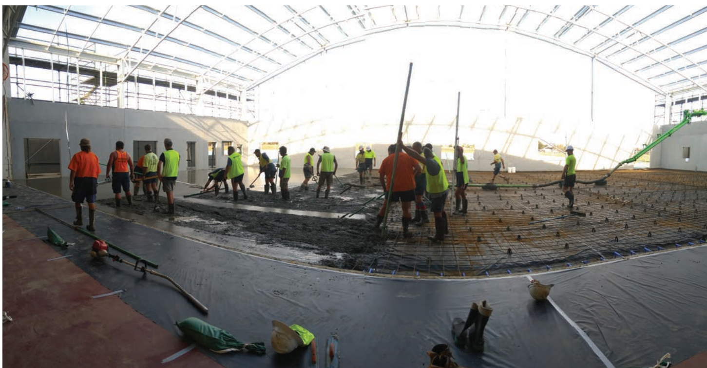
ABOVE: Concrete being poured for the Sports Dome extension.
