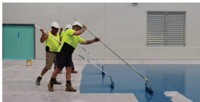
ABOVE: The specialised flooring being applied inside the Sports Dome in late December 2018.
